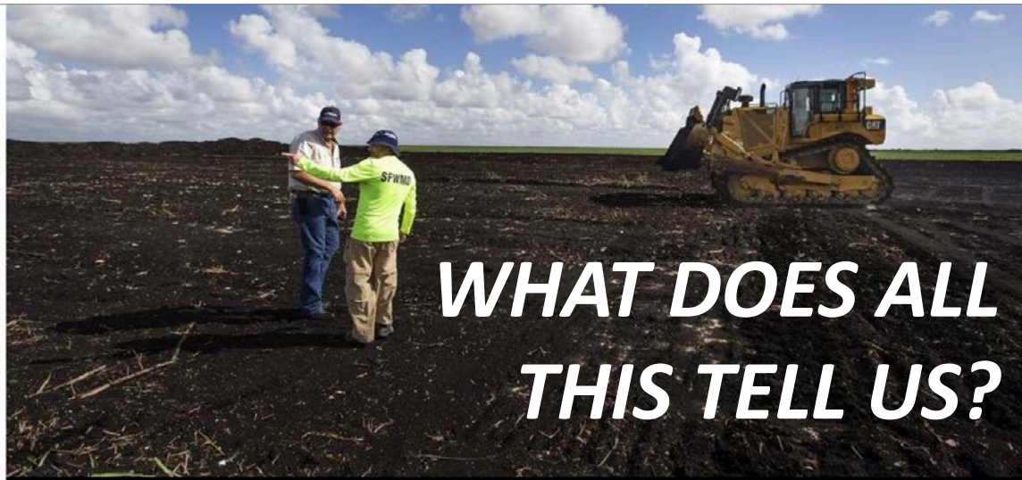
South Florida Water Management District has begun clearing a sugar cane field to make way for a reservoir south of Lake Okeechobee to hold overflow releases. Muck is being scraped away to the capstone for materials to be stored on in preparation for the beginning of construction. [ALLEN EYESTONE/palmbeachpost.com]
